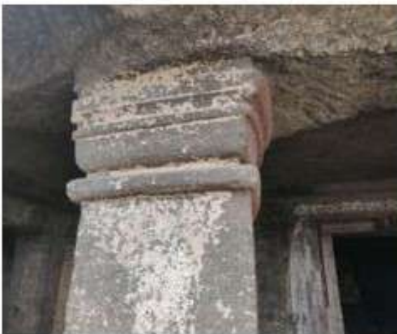
Pillar of Nagarjun cave
